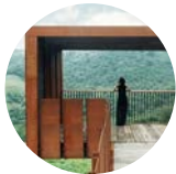
Iconic Infrastructure to showcase the location of the biggest alluvial nugget at Welcome Stranger site.
