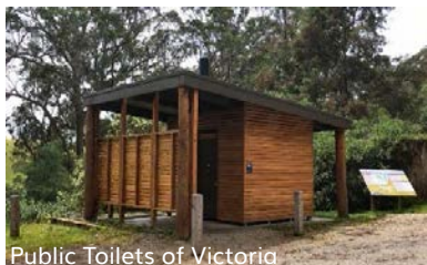
Public Toilets of Victoria Agnes Falls, Gippsland
