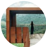
Iconic infrastructure to showcase the Balaclava open cut mine as a spectacular example of early quartz reef mining at Whroo Historic Reserve.
